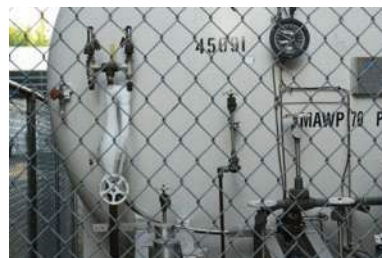
Difficult inspection sites
